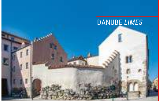
Above: Parts of the Roman wall at the north-eastern corner Below: The "document Legionslagermauer" at Dachauplatz
